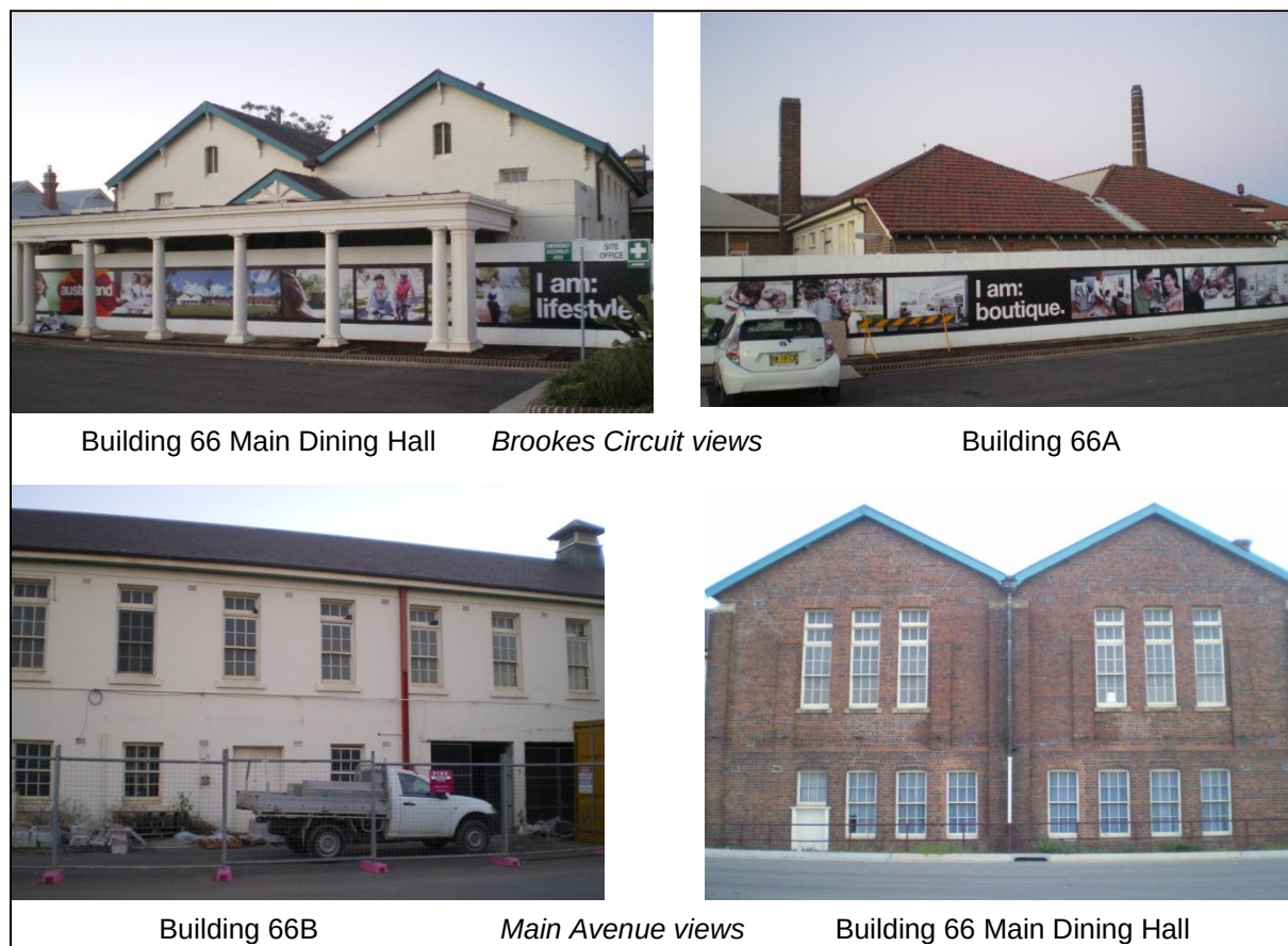
Figure 3: Views of Building 66
